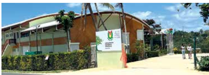
The new Foundation Building of the National University of Vanuatu
